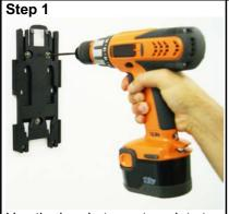
Use the bracket as a template to mark the mounting hole pattern. Drill the hole for the supplied 1/4" anchors and secure the bracket with the three supplied screws.
